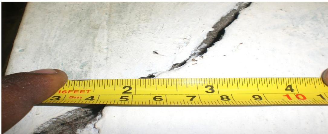
**Fig.5. Measurement of inclined cracks**
