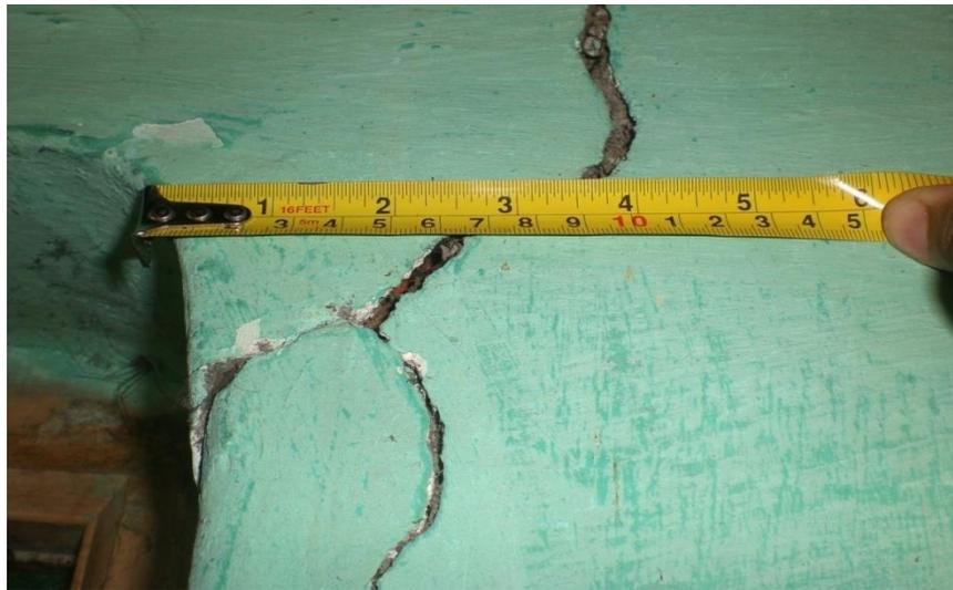
**Fig.4. Measurement of cracks**
