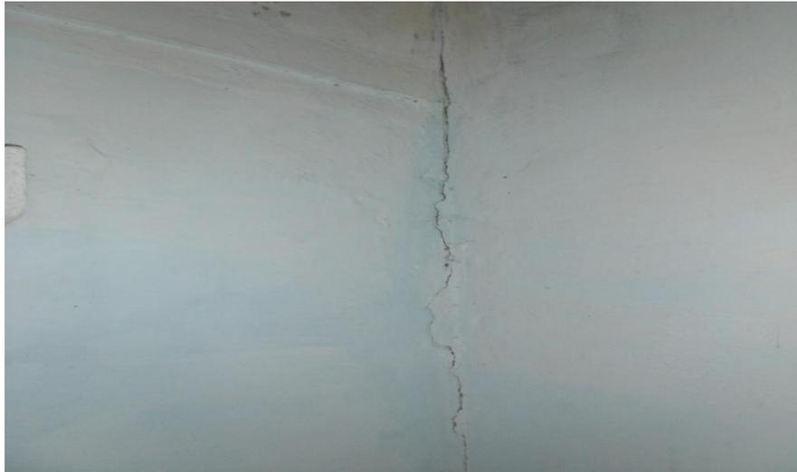
**Fig.3. cracks at wall junction**
