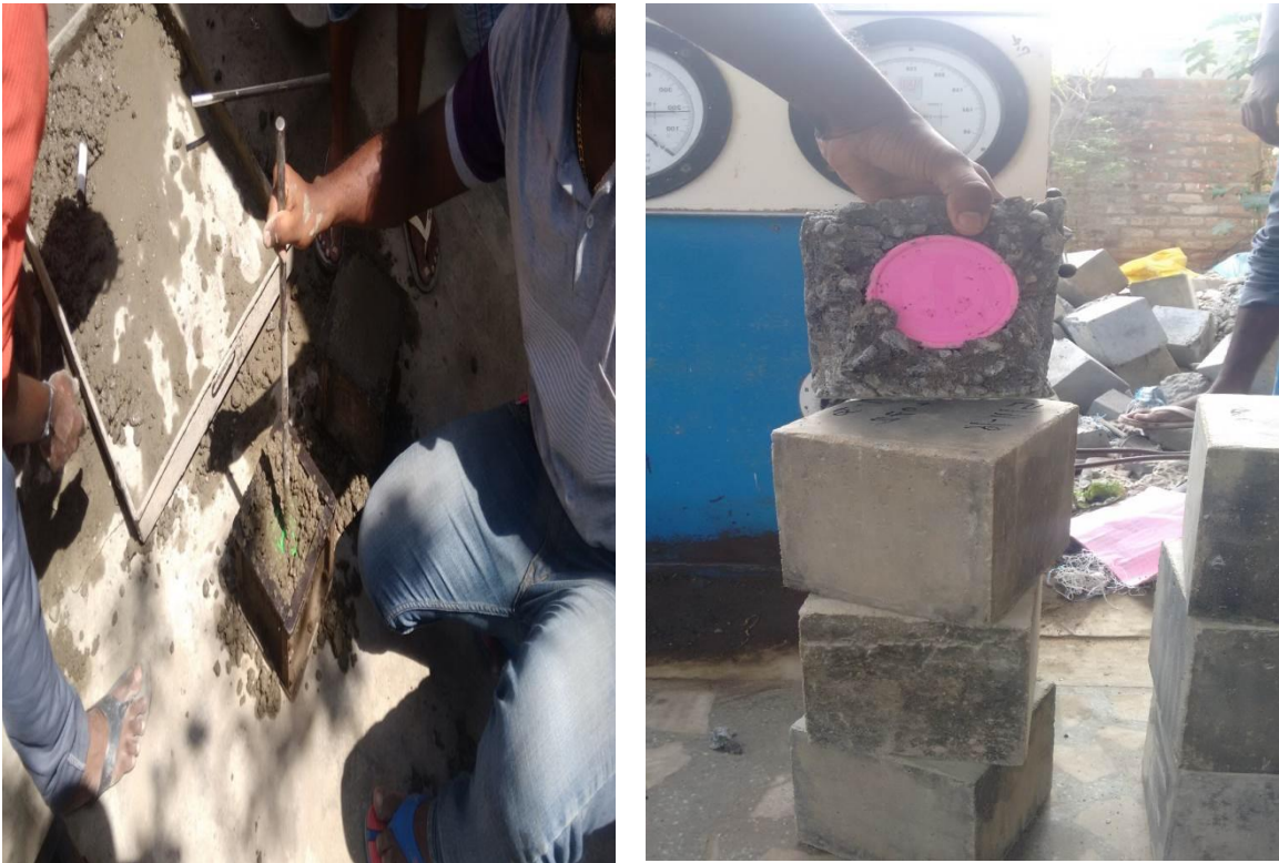
Fig No: 2 Casting of Cubes
