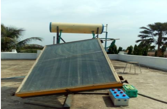
Figure 1 Position of the panel at 3.00 pm
