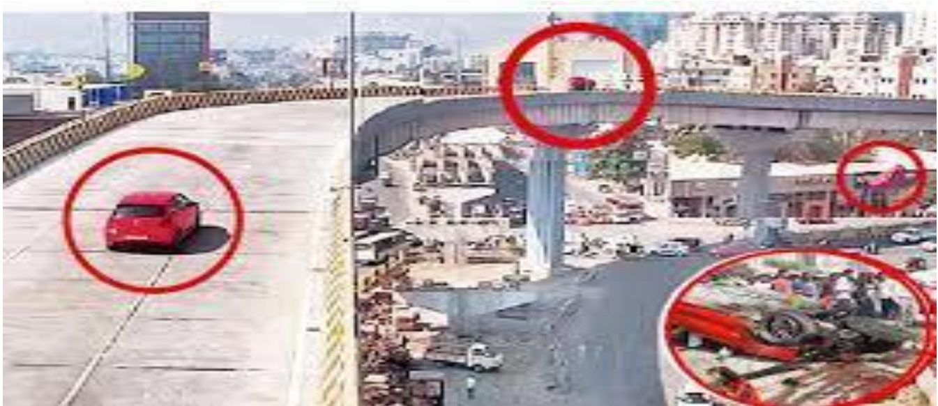
Figure 1: Car falling down from the Flyover
