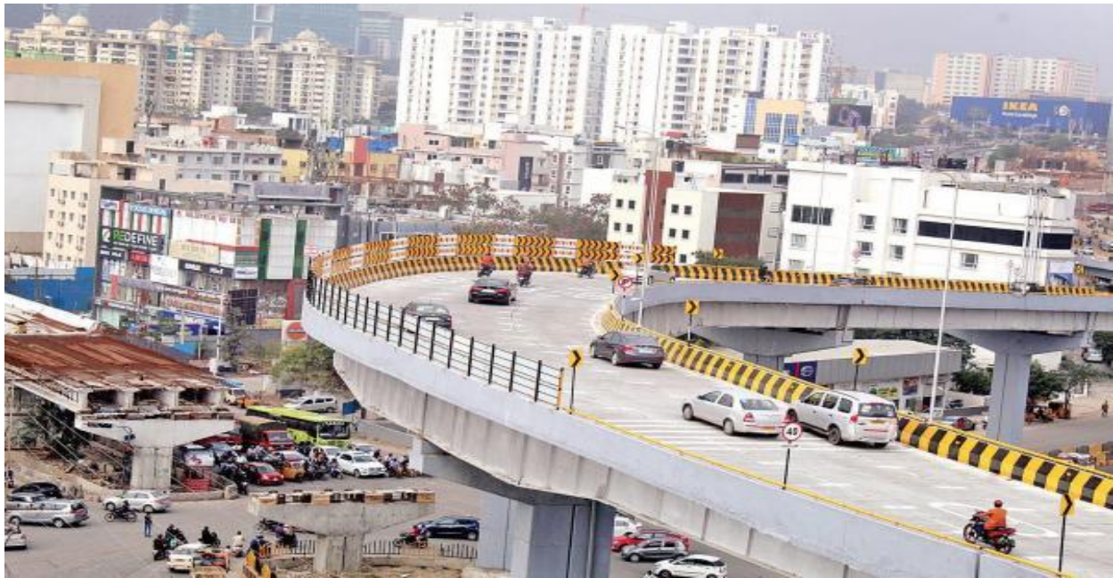
Figure 3: Side barriers/rollers installed all over the flyover after the incident
