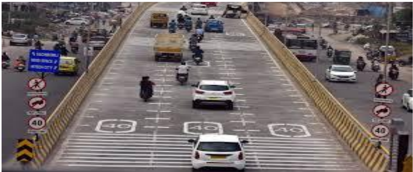
Figure 4: Rumble strips and sign boards were installed after incident
