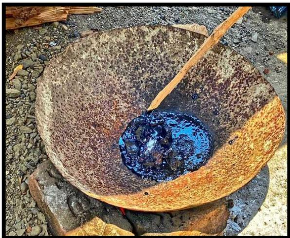
Figure 1: Melting of Bitumen
